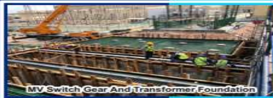
MV Switch Gear And Transformer Foundation
