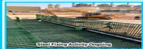
Steel Fixing Activity Ongoing
