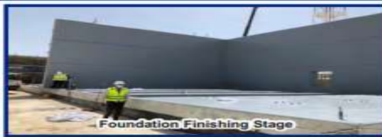
Foundation Finishing Stage
