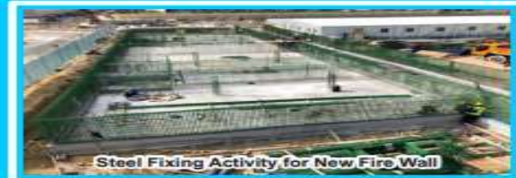
Steel Fixing Activity for New Fire Wall
