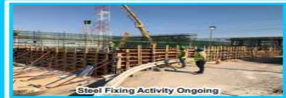
Steel Fixing Activity Ongoing
