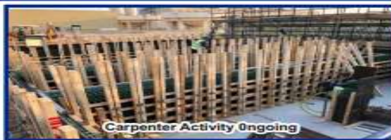
Carpenter Activity Ongoing
