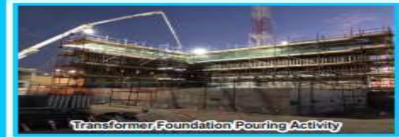
Transformer Foundation Pouring Activity
