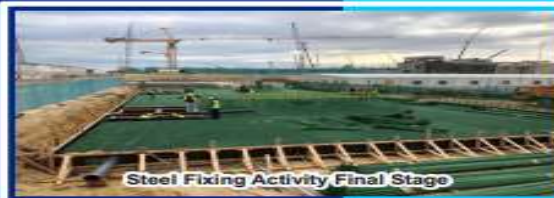
Steel Fixing Activity Final Stage
